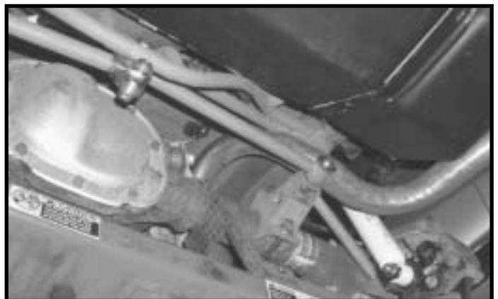
Figure 6.1 - Final installation Passenger side.
