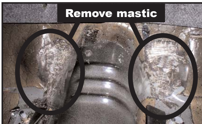
Figure 1.0 - Remove floor mastic.
