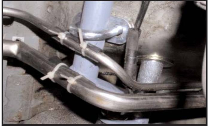
Figure B - Brake/Fuel lines with protective sleeve.
